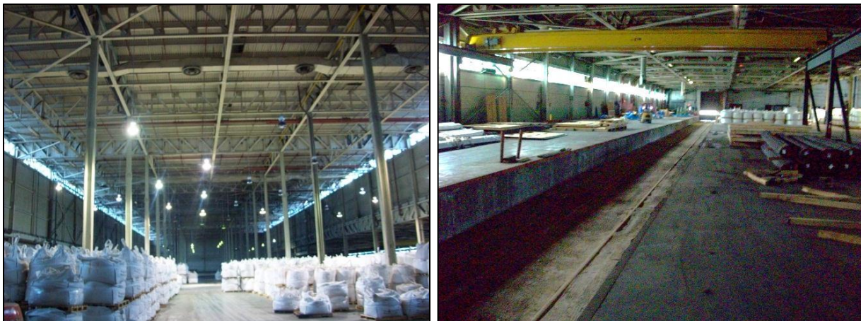
Figure 13: Storage at the Euclid Facility and Interior Rail Unloading Area
