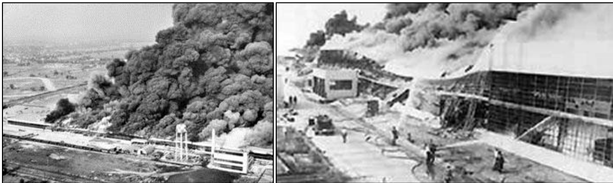
Figure 3: 1957 Fire at the General Motors Hydra-Matic Facility
