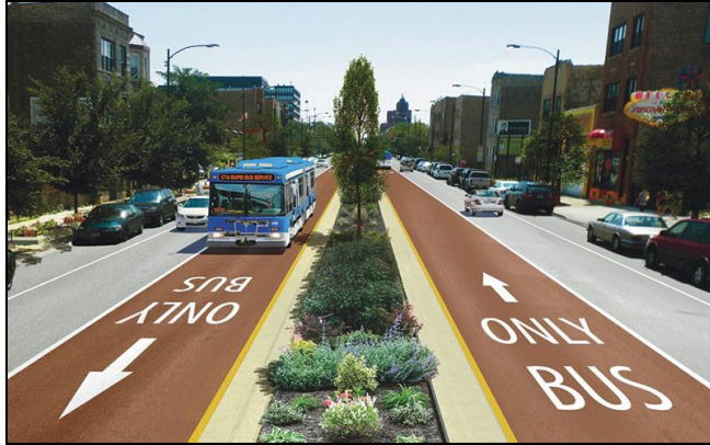
FIGURE 5. BUS RAPID TRANSIT INFRASTRUCTURE 57
