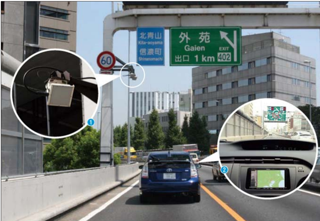
Figure 11: ITS Spot Service in Japan Source: Japan 2012
