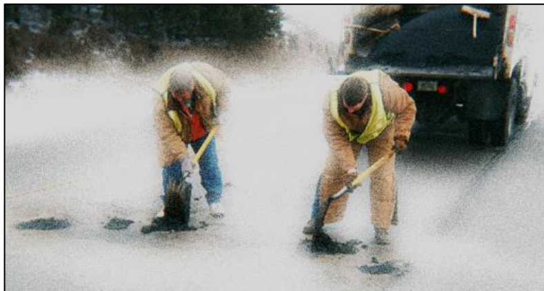
FIGURE 14: MAINTENANCE CREWS PERFORM BOTH REACTIVE AND SCHEDULED MAINTENANCE
